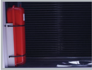
closed expansion tank
